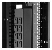
The optional power strip mounting bracket mounts vertical power strips without taking up valuable U-space.
